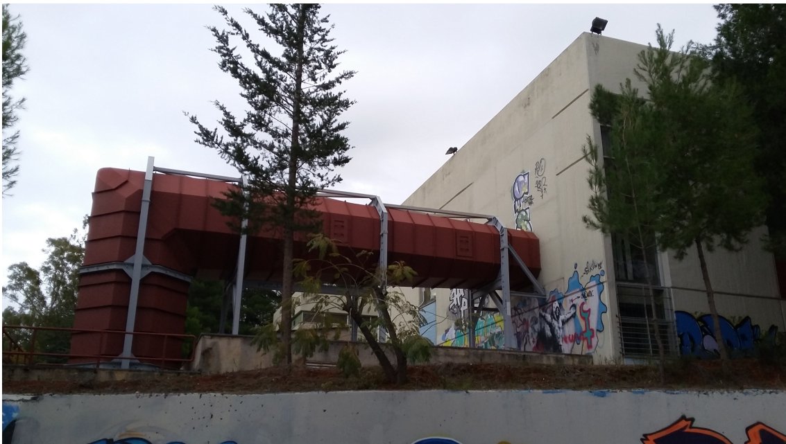
Figure 7.4: The exterior section of the wind tunnel
